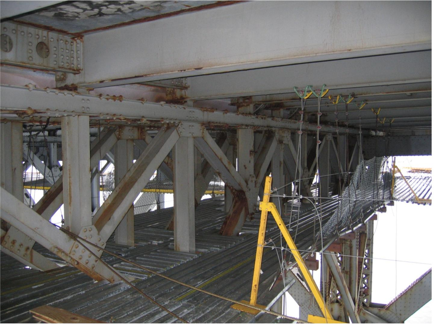
**East Deck Truss – Cable Supported/Metal Deck Platform System At Expansion Joint**
