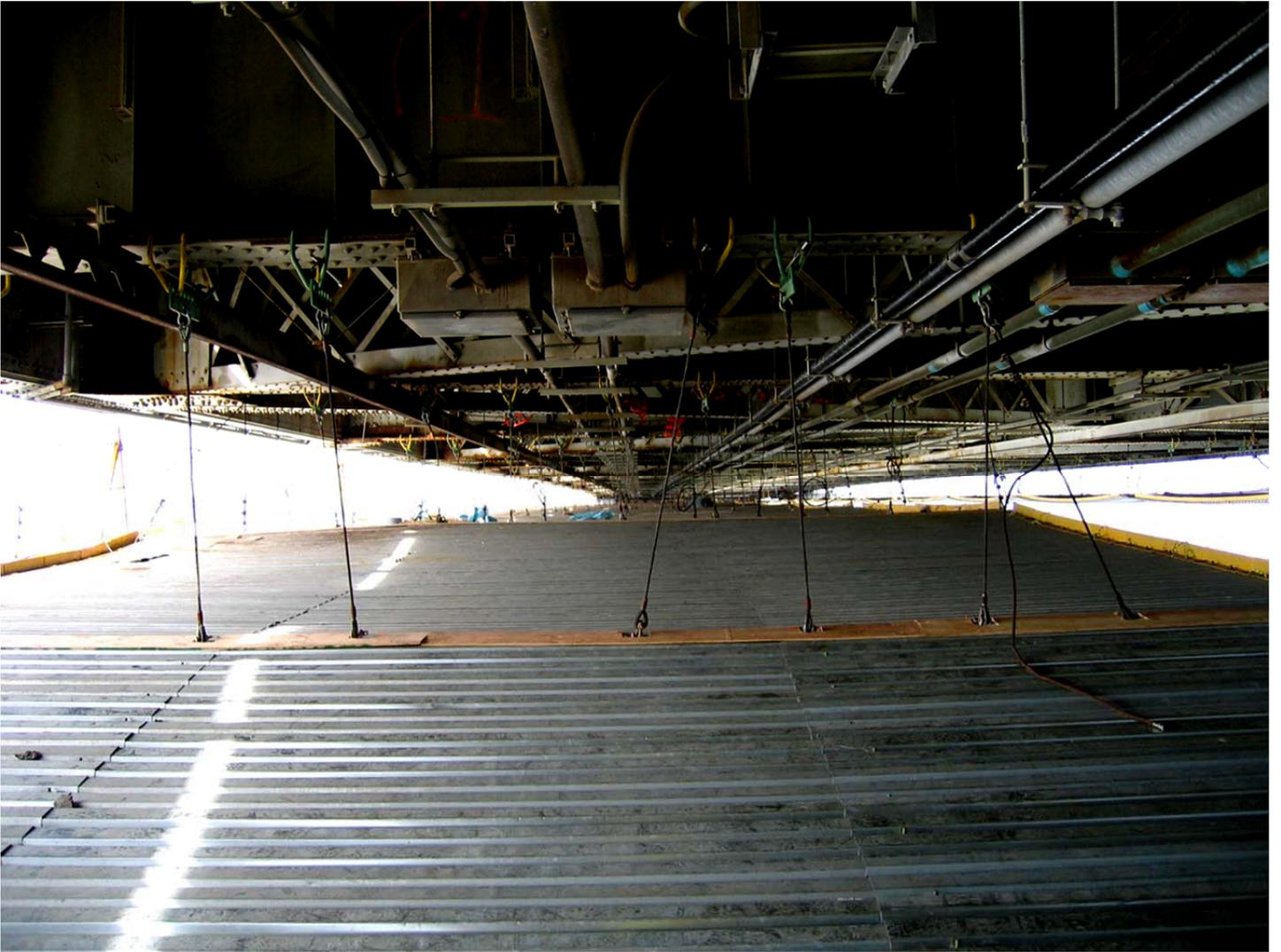
**Main Span-Cable Supported/Metal Deck Platform System w/Plywood Closure Strips**
