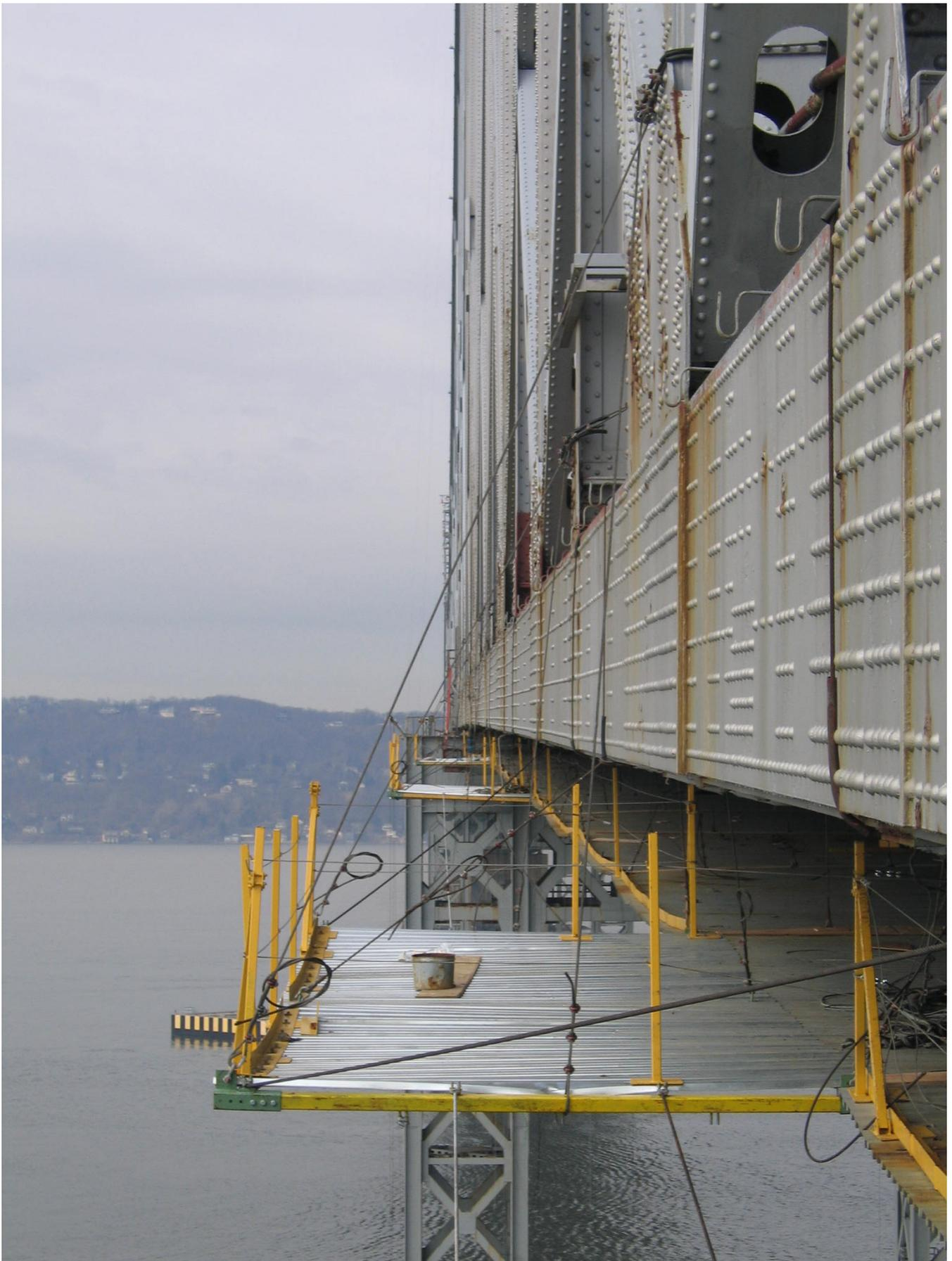
**Main Spans -Cable Supported/Metal Deck Platform System
