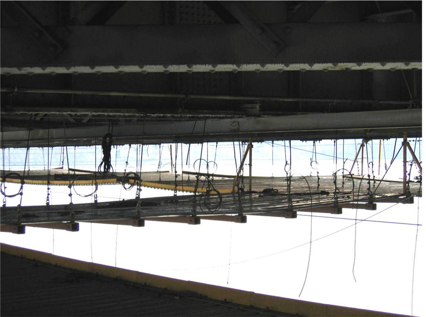
**Tube Supported Cross Over Platform Installation Between N & S Main Platforms**
