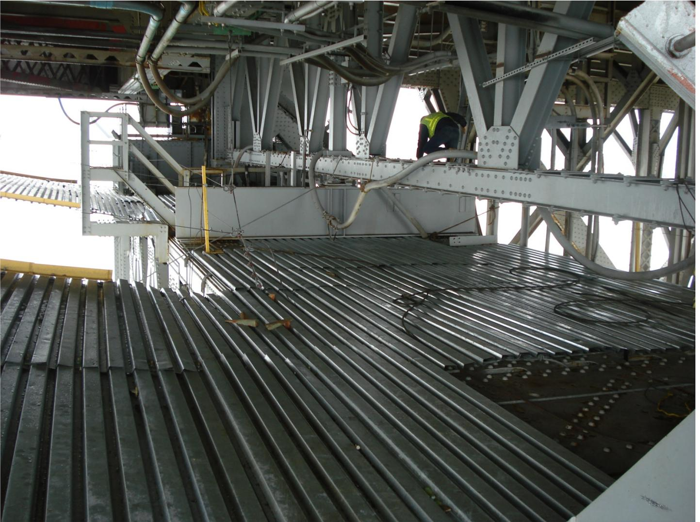
**Main Spans, Cantilever & Anchor Spans Cable Supported/Metal Deck Platform System
