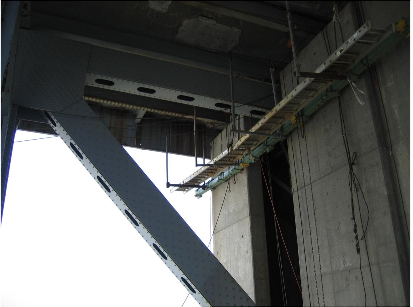
**East Deck Truss – Concrete Pier – Horizontal Support Beam Assembly
