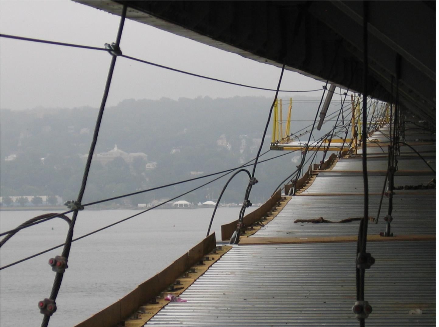
**East Deck Truss – Cable Supported/Metal Deck Platform System
