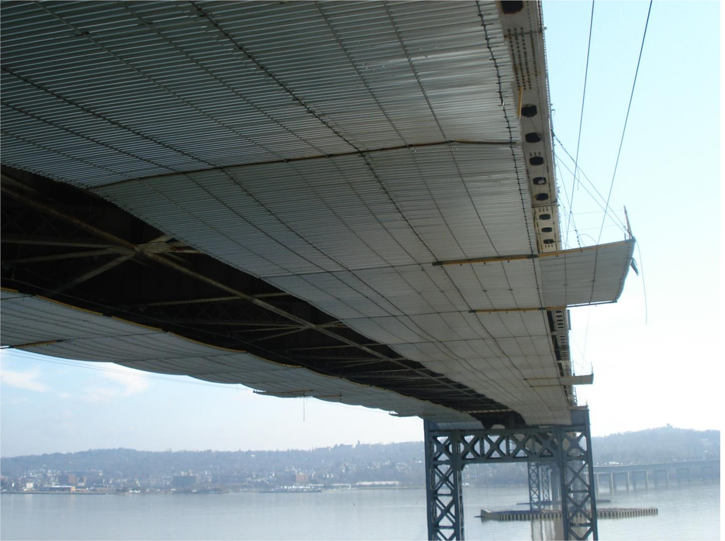
**Main Spans -Cable Supported/Metal Deck Platform System
