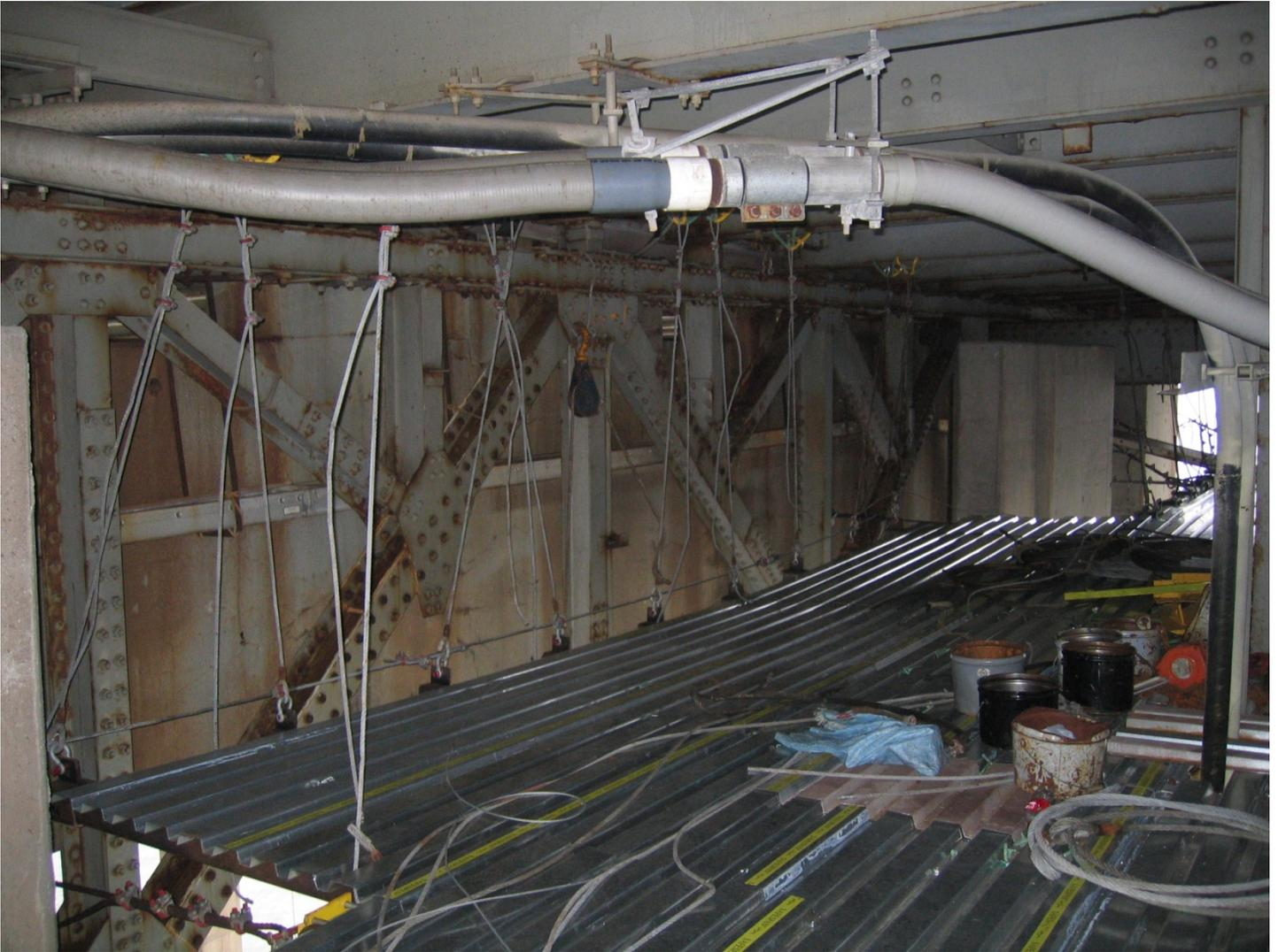
**Cable Supported/Metal Deck Platform East Deck Truss – At East Concrete Pier**
