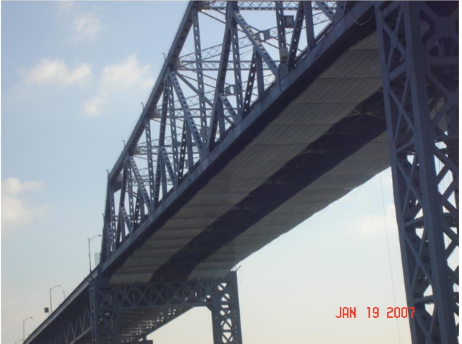
**Anchor Span -Cable Supported/Metal Deck Platform System**
