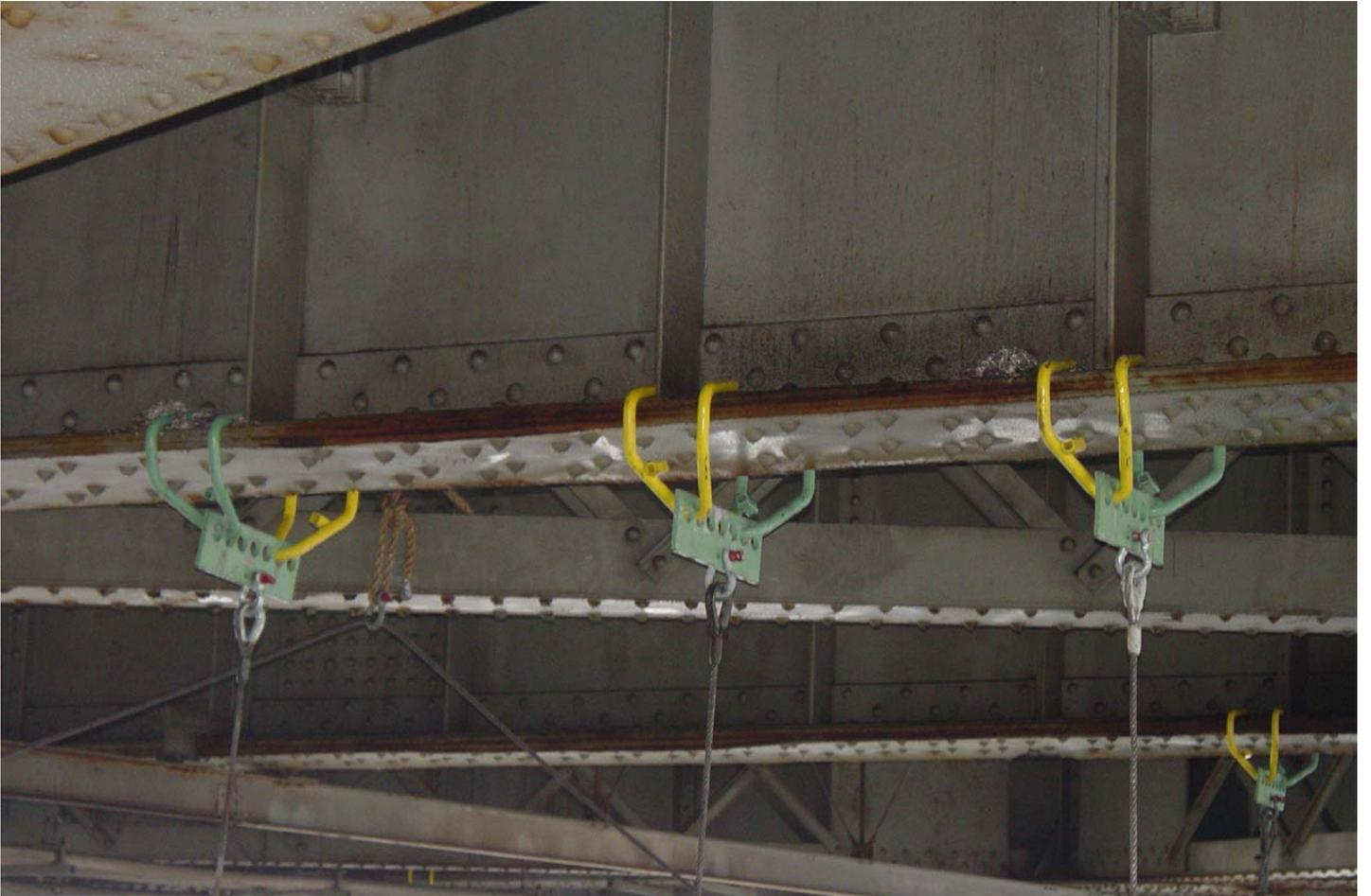
**Beam Flange Clamp Hanger Assemblies & Vertical Cable Tie Ups**
