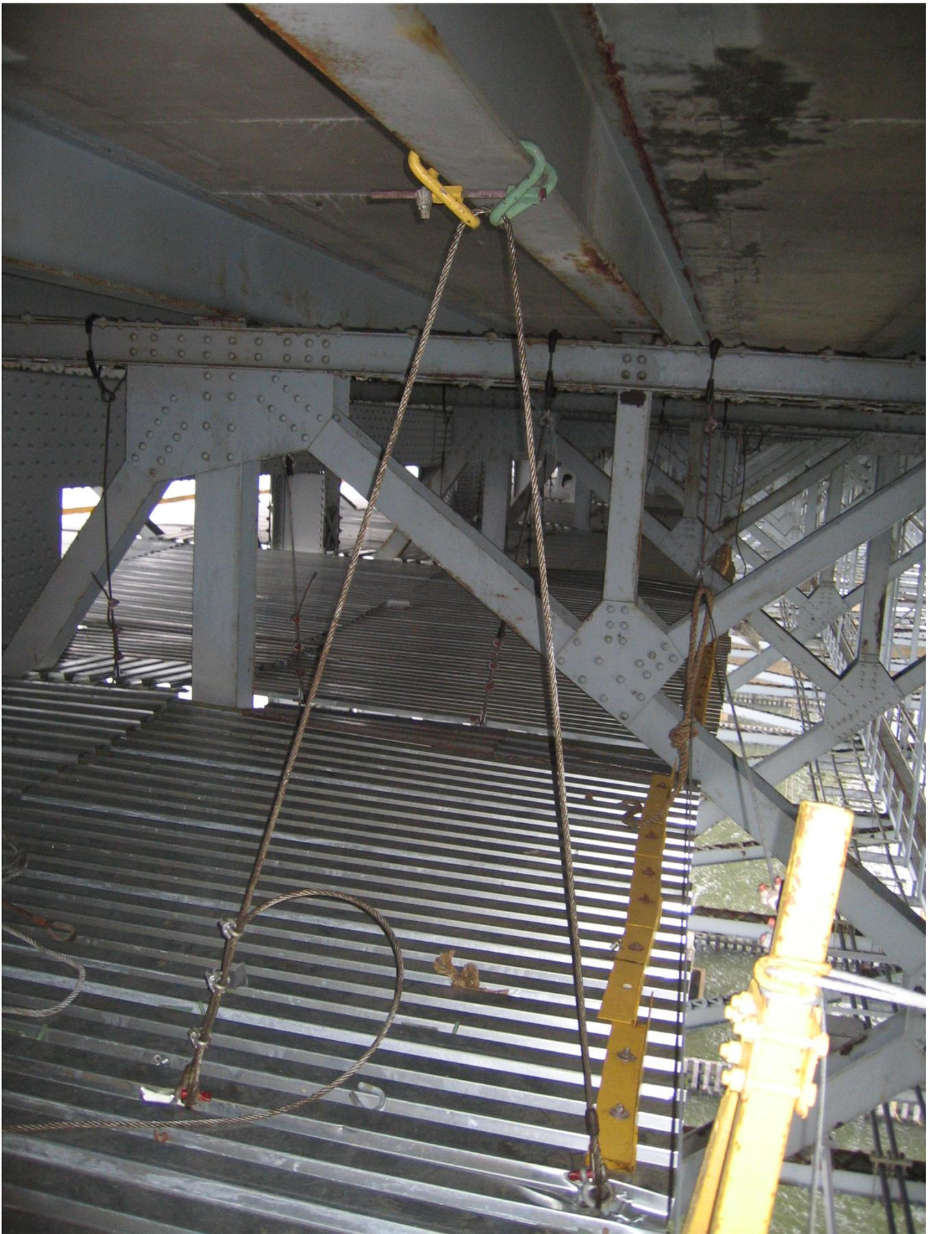
**East Deck Truss – Cable Supported/Metal Deck Platform System**
